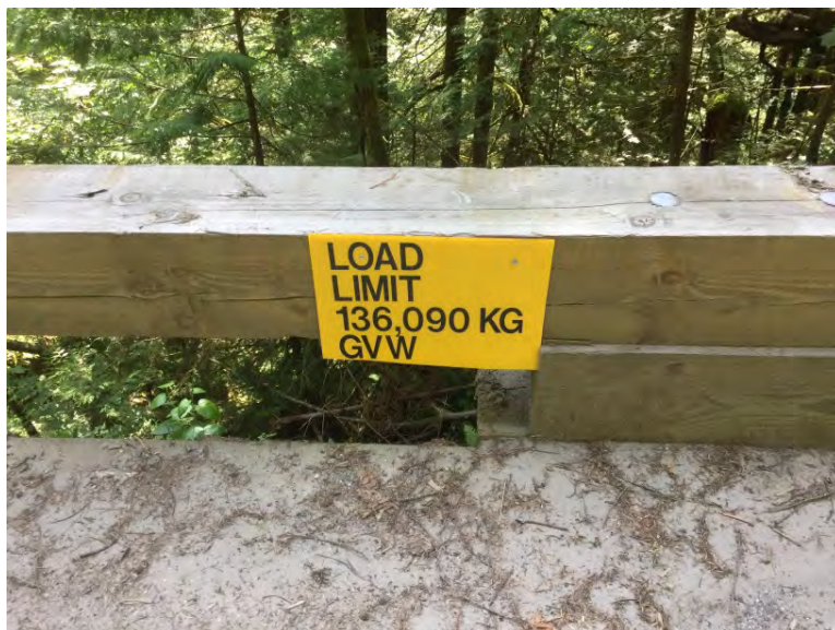
Load Rating Sign
