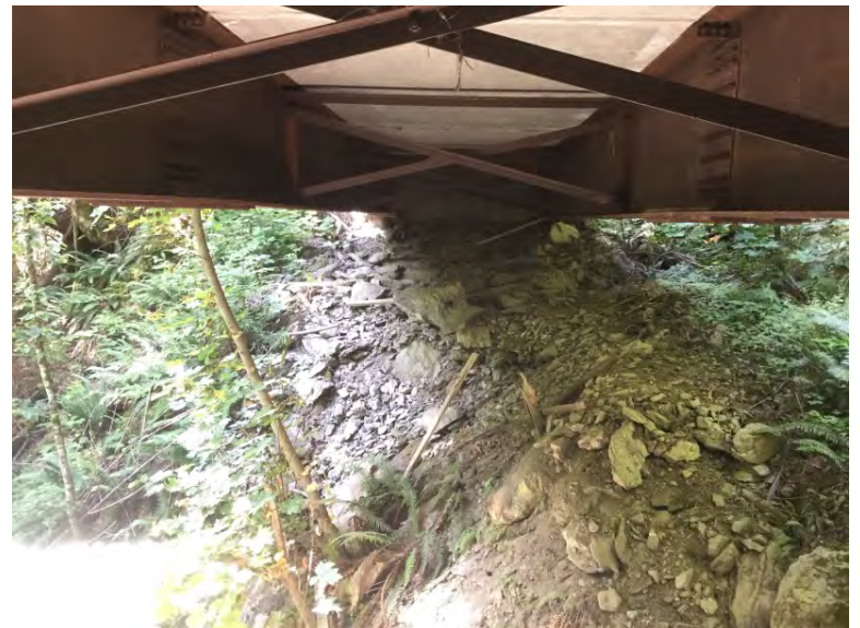
Right Bank Abutment when facing downstream
