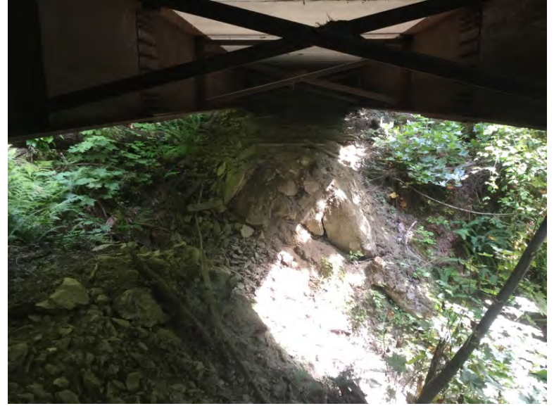
Left Bank Abutment when facing downstream
